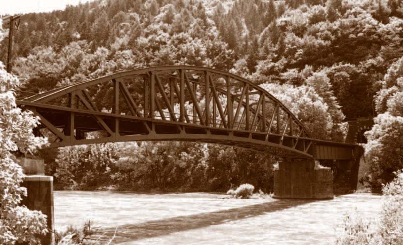
One of the two bridges at Strečno.
