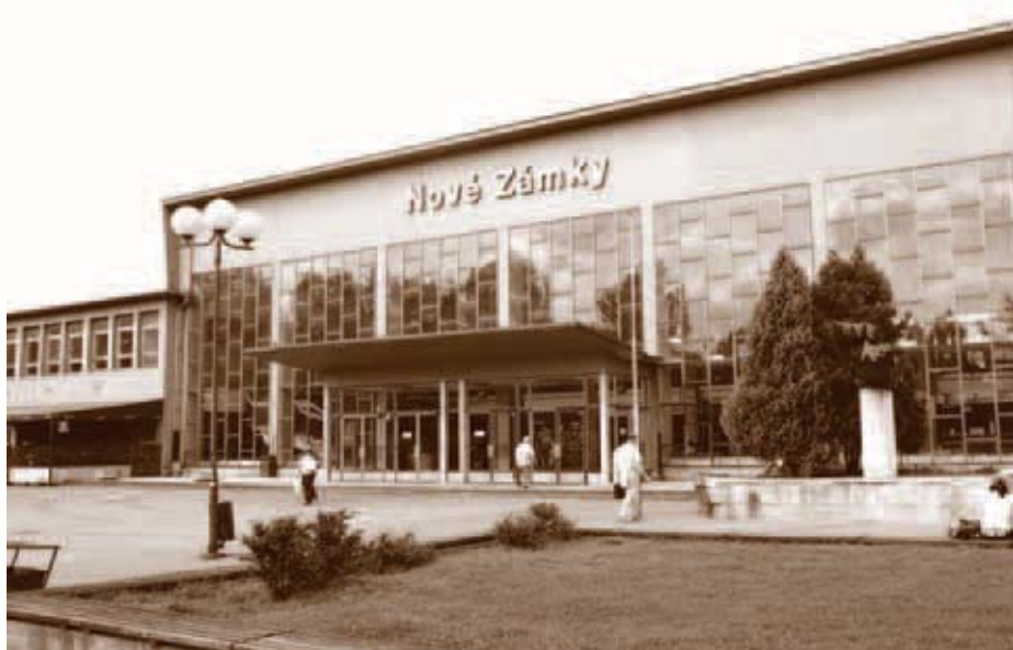
View of Nové Zámky station from the town.
