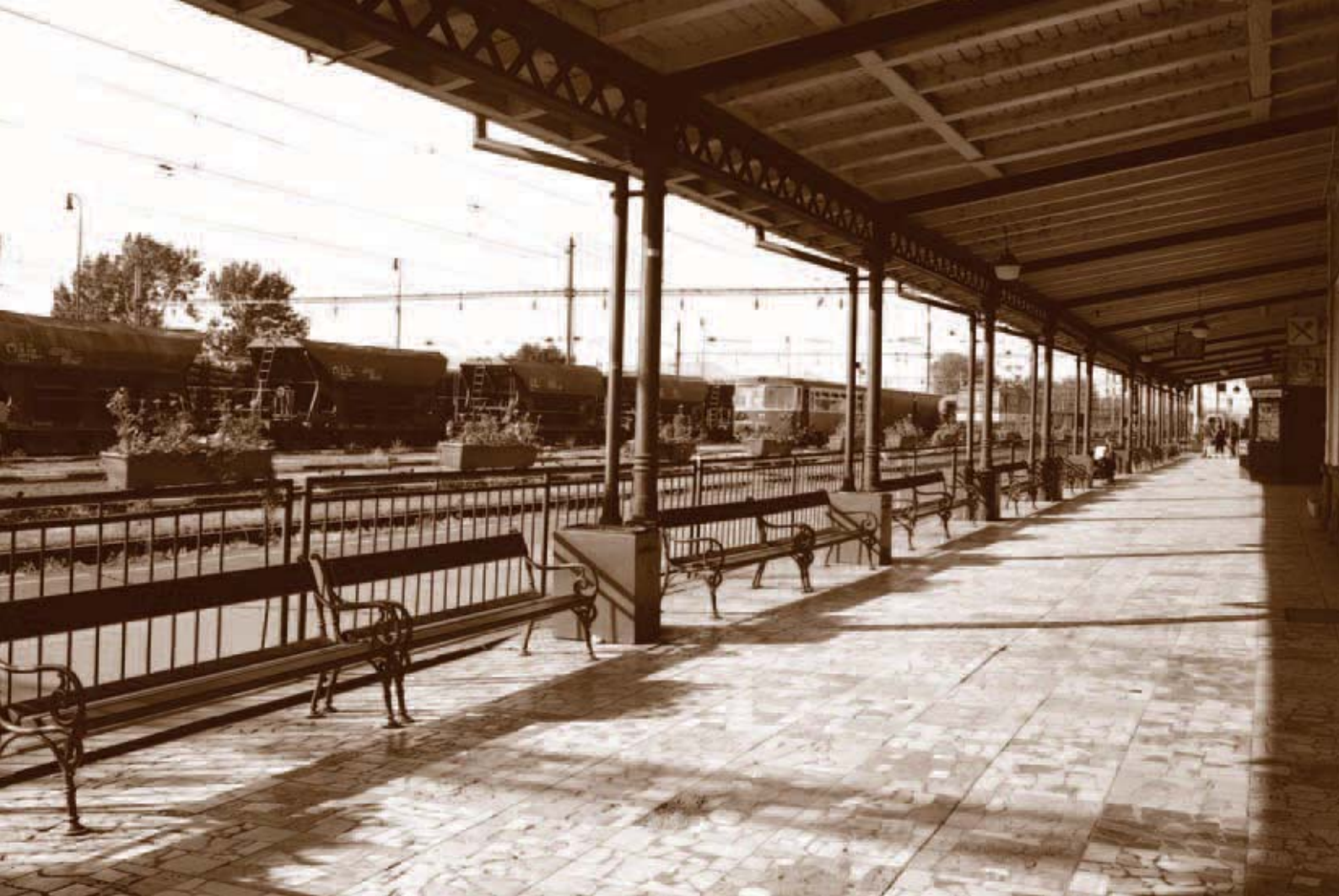
A platform at the railway station in Trenčianska Teplá.
