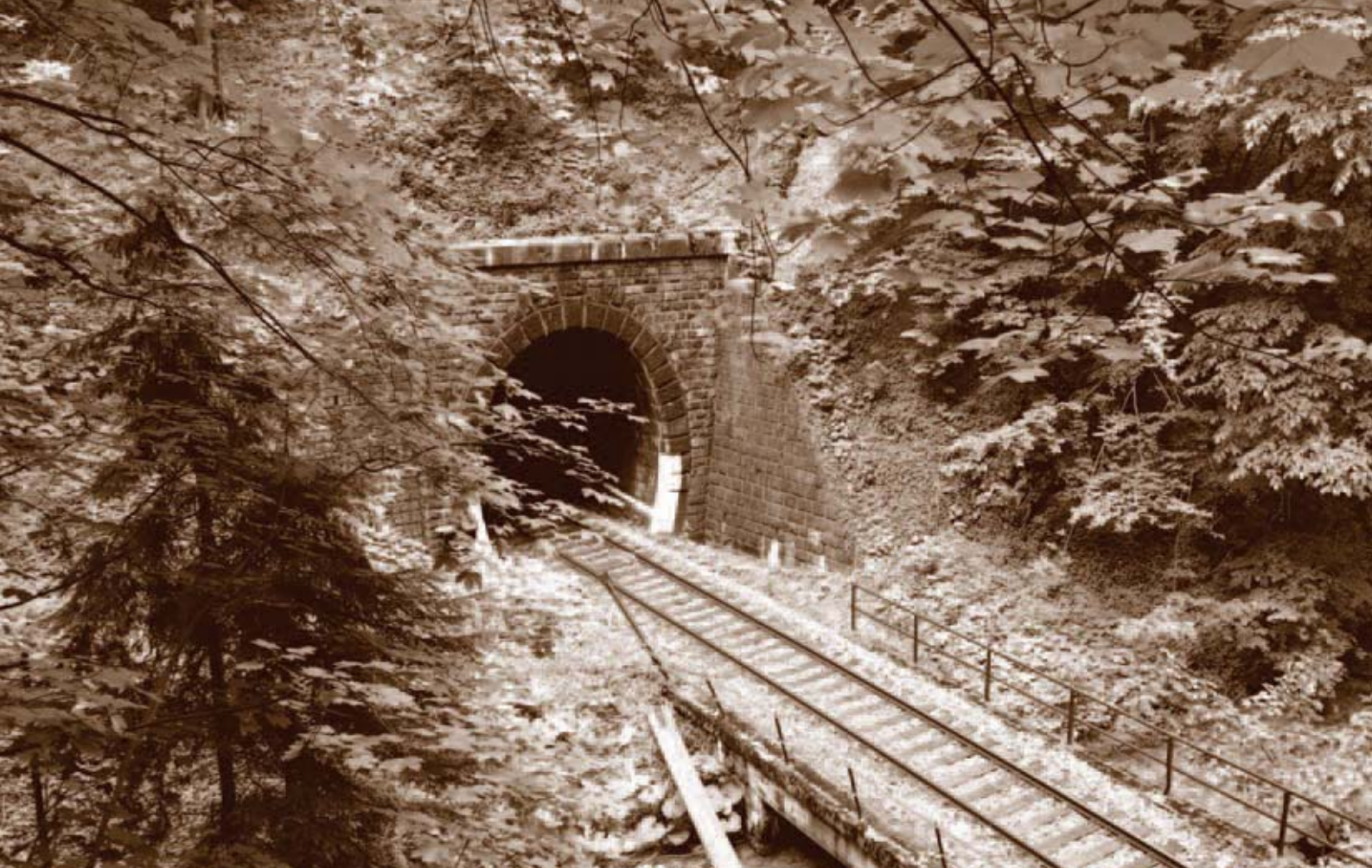
Two man-made constructions, a tunnel and a bridge, on the SNP tracks between Banská Bystrica and Horná Štubňa.
