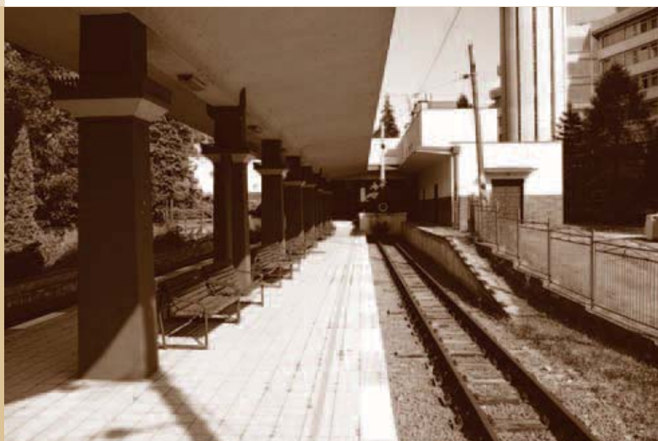
The railway station in Trenčianske Teplice - view from the platform.
